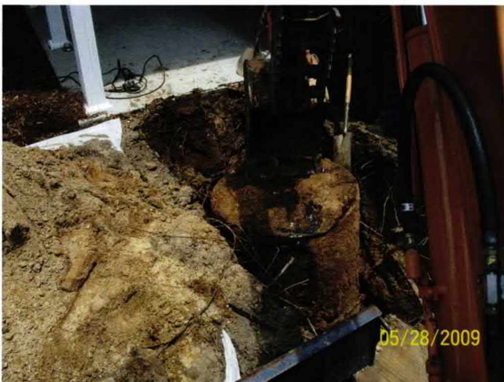
Picture 2: UST 1047Gardenia during removal.
